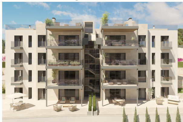
Frontal view of building
