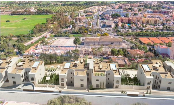
Santa Ponsa New Built
