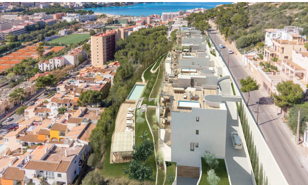
Santa Ponsa New Built
