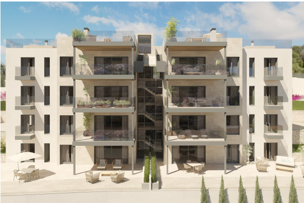
Frontal view of building
