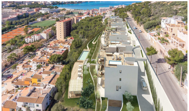
Santa Ponsa New Built
