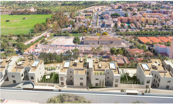
Santa Ponsa New Built
